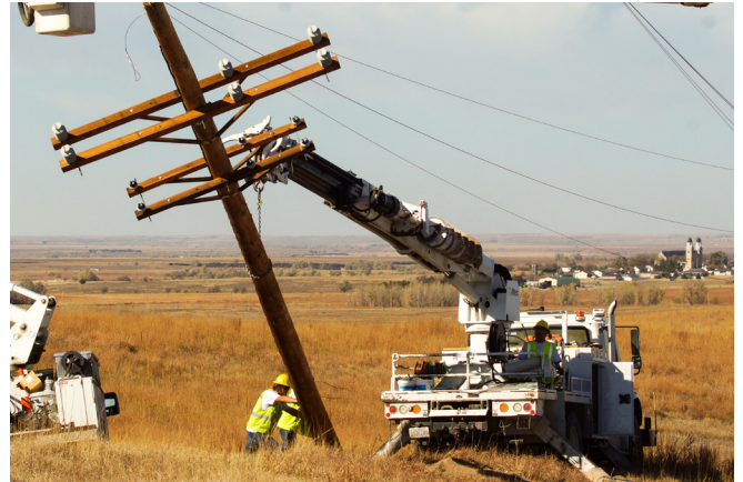
The digger trucks are used to raise the new pole into the hole that has been drilled. Chains are used to lift the pole until it is high enough for the digger to grab it. Lineworkers pull the wires back to give room for the installation.
