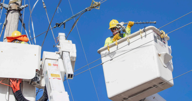
A junction pole requires additional equipment and set-up. On the right, Jacob is preparing a “dead-end shoe” to attach to the pole and firmly hold the end of the wire.
