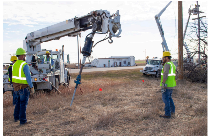
The digger truck is using a Kelly bar to spin an anchor into the ground which will hold the guy wires that keep the pole secure. Jeremy is running the controls while Keath, Garrett and Austin help monitor for correct placement. They use hand signals to communicate with the operator.
