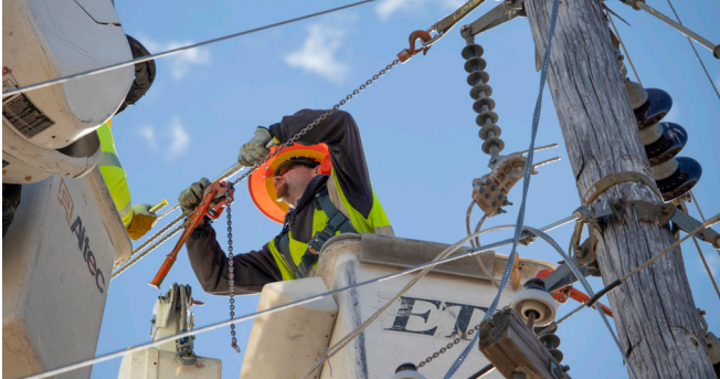
The new pole would be relocated several feet away, so the lines had to be longer. Brett is using an aluminum “quick sleeve” to splice together more line.
