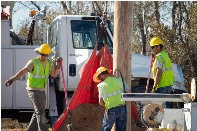
Crew members are refilling a hole around a pole that has been set. Jameson and Cory are shoveling the dirt off the blanket into the hole. Jeremy is using a hydraulic tamper to pack the dirt tight and keep it from settling. He will do this each time more dirt is added.
