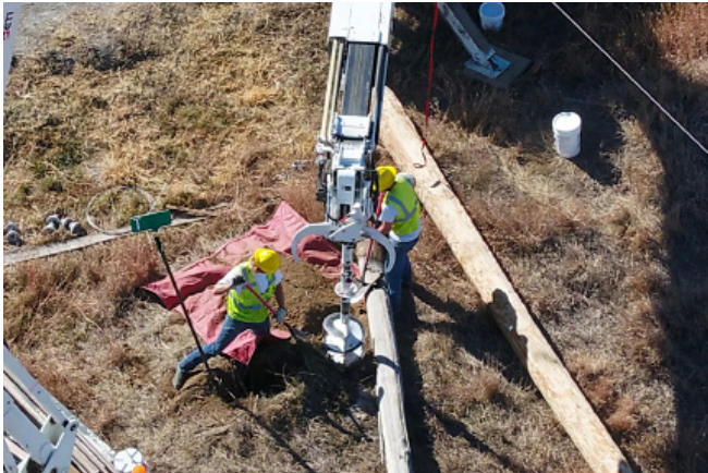
In this case, the new pole will go in the same hole as the old, but the auger is drilling a bigger hole since the new pole is larger. Extracted dirt is collected on a red blanket that keeps it out of the grass. Later, it attaches to the digger truck to help with the labor when it's time to refill the hole.
