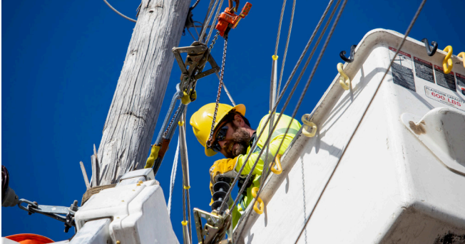
Insulators come in many shapes, sizes and materials. For this project, the old porcelain bell insulators are being replaced with epoxy insulators that are made of fiberglass and covered in rubber.
